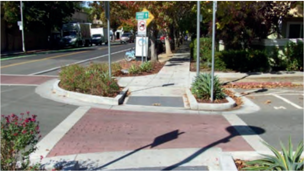
Figure A8. A pedestrian bulb-out reduces the number of lanes one has to cross, while also increasing their visibility at the intersection to oncoming vehicles (Institute of Transportation Engineers, n.d.).
