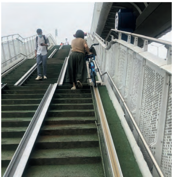
Figure A26. Wheel ramp in Beijing, China, allow seamless integration from ground-level to elevated cycle highway (ITDP, 2021).
