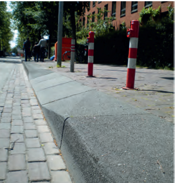
Figure A11. Bollards at the curb cut prevent vehicles from entering the sidewalk and disrupting the pedestrian environment (Foletta & Henderson, 2017).
