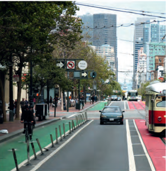
Figure A12. An on-street bicycle lane that is painted green and separated from the vehicle lane with flexible soft hit posts (Foletta & Henderson, 2017).
