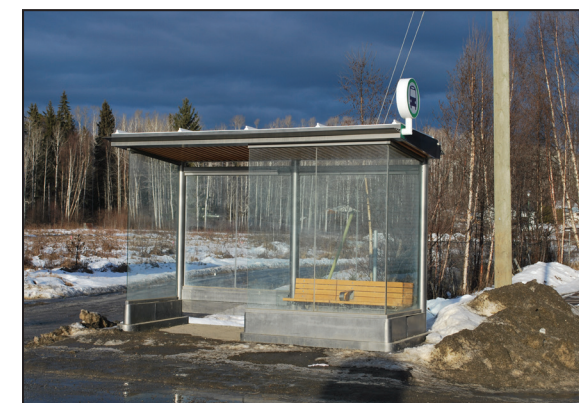
Figure 11: Upgraded bus stop - BC Transit. Photo Credit: SCARP Planning Studio
