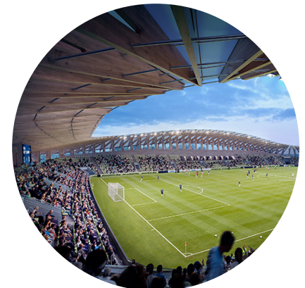
The New Lawn timber-built stadium in Nailsworth, England
