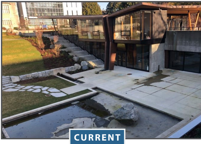
Area 7 - The Bowl: Engineered Detention Pond (Gravel)
