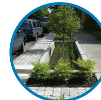
Stormwater Tree Trenches
