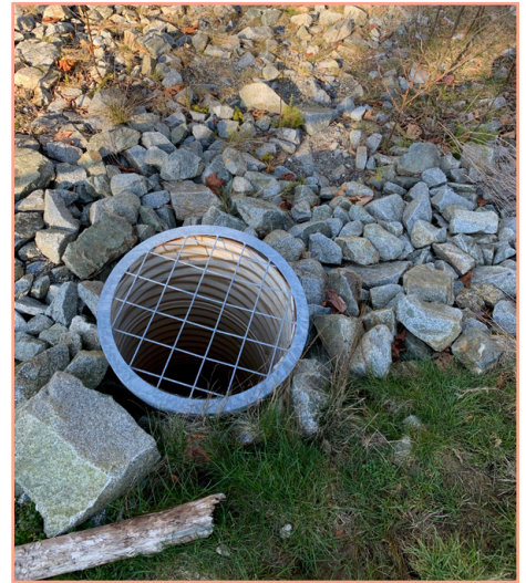
Figure 24. Feature of the existing crossing on the site.
