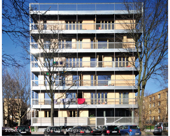
Figure 6. R-50 Housing Project, Berlin
