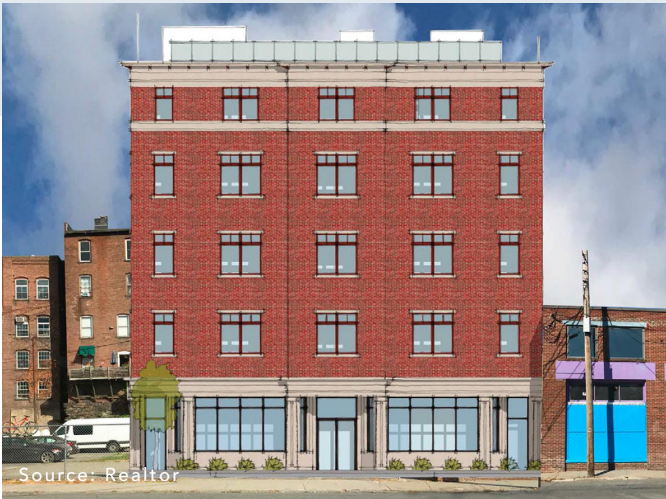
Figure 20. Wilder Block. Windham & Windsor Housing Trust
