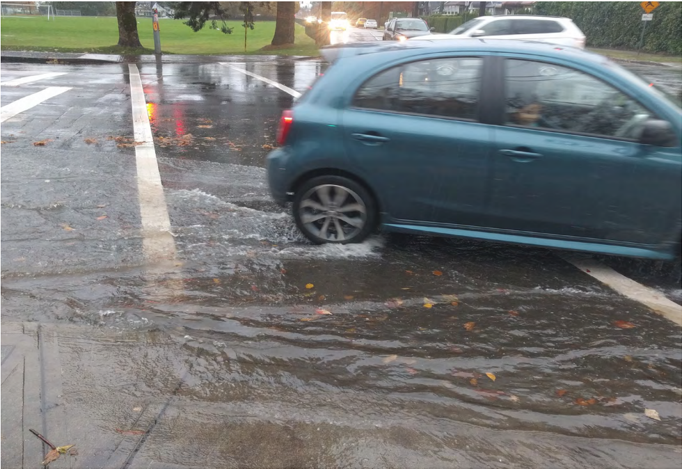
Instance of heavy ponding on the intersection of 8th St & 8th Ave
