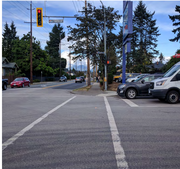
The curb letdowns on the east side of the intersection are not ideal (south-east pictured here). The crosswalks are worn
