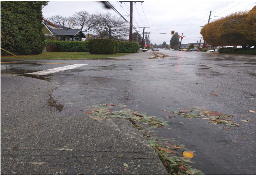
Instance of ponding on the intersection of 10th St & Kingston St
