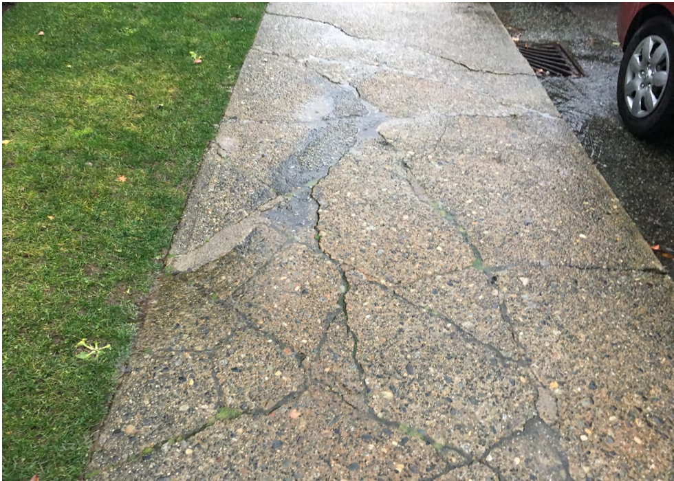
Extended damage of the sidewalk, leading to uneven surface in a high senior pedestrian traffic location right outside the Century House on 8th St
