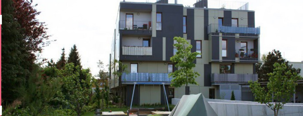
Figure 3. [ro*sa] 22 building (Cohousing Cultures, 2018)
